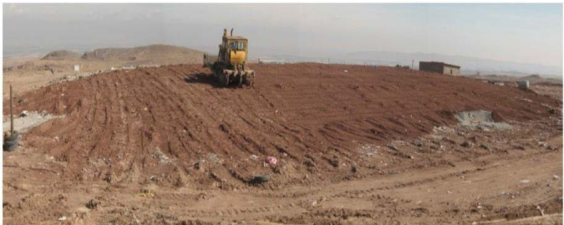
Figure 7.13: Implementation of Final Cover for Tehran Pilot Scale Landfill
