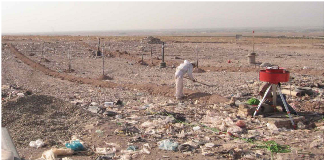
Figure 7.19: Placement of HDPE Pipes for Profiler and the Fixed Extensometers in Tehran Pilot Scale Landfill
