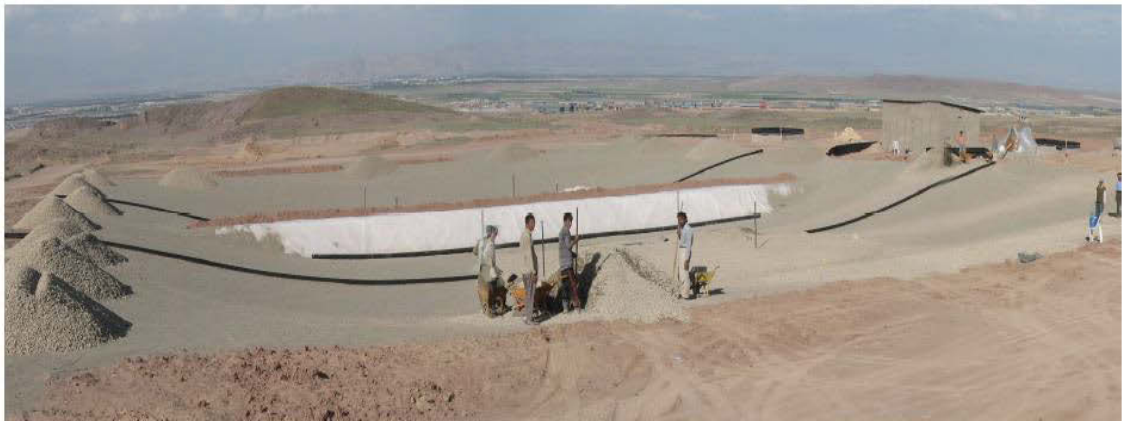
Figure 7.11: Construction of Tehran Pilot Scale Landfill
