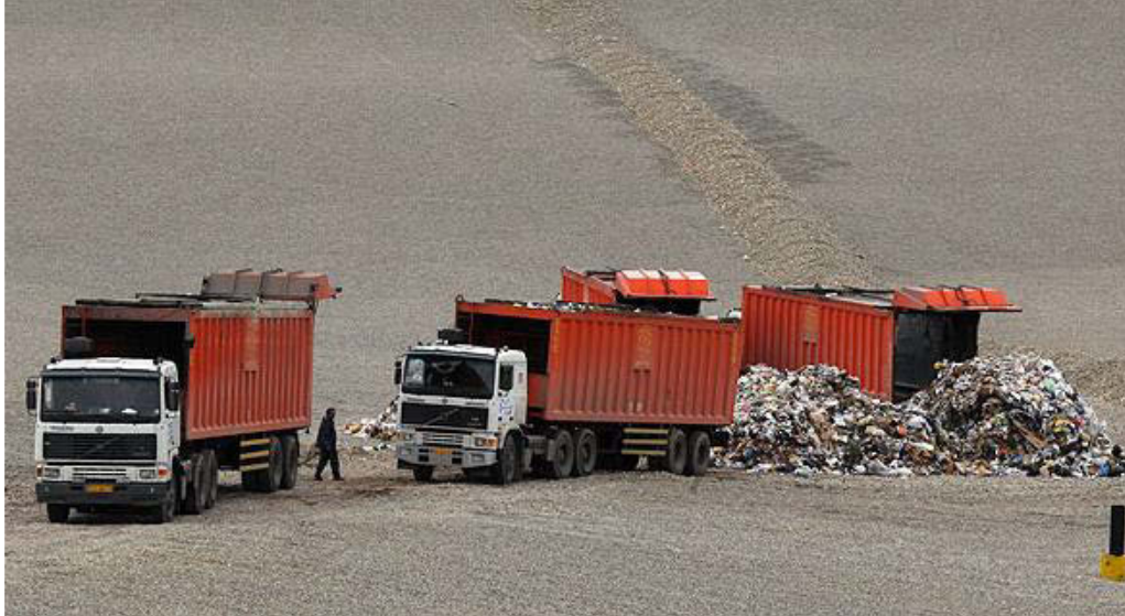
Figure 7.9: Drainage Layer Implementation and Waste Disposal in Tehran Sanitary Landfill (Photo Taken by the Author)
