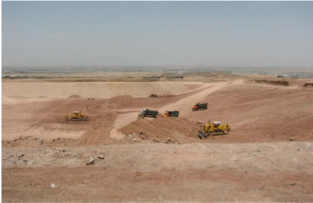
Figure 7.5: Excavation Phase of Tehran Sanitary Landfill (Photo Taken by the Author)
