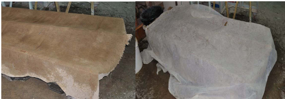
Fig. 3.4: Covering concrete specimens after casting with wet burlap (left) and polyethylene sheet on top of the burlap (right)
