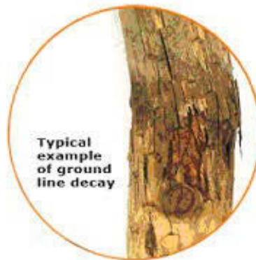
Figure 6-7 Typical example of ground line decay
