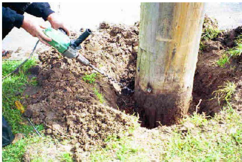
Figure 2-2 Inspection below ground line (Ausgrid, 2006)
