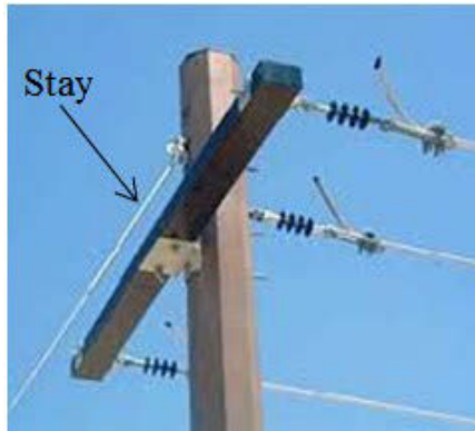
(a) Stay applied at the termination of distribution network
