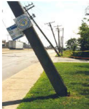
Figure 6-4 Collapse of timber utility poles
