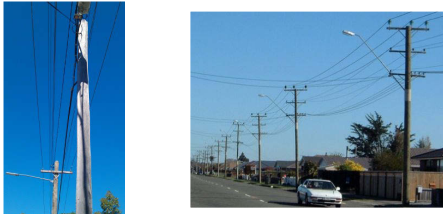
Figure 6-2 Cables attached to timber utility poles for network distribution
