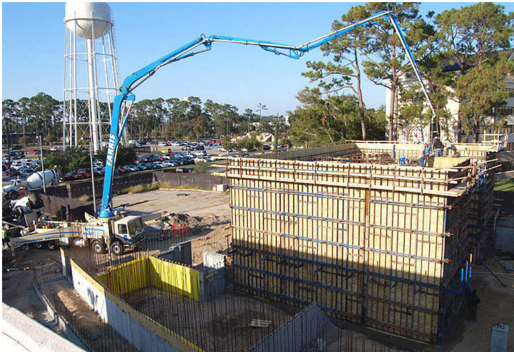
Figure 1.4 Construction Site with a Concrete Pump Truck
