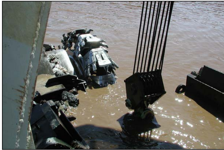
Figure 5.57: View of suction-cutter dredge head raised from the water for maintenance.
