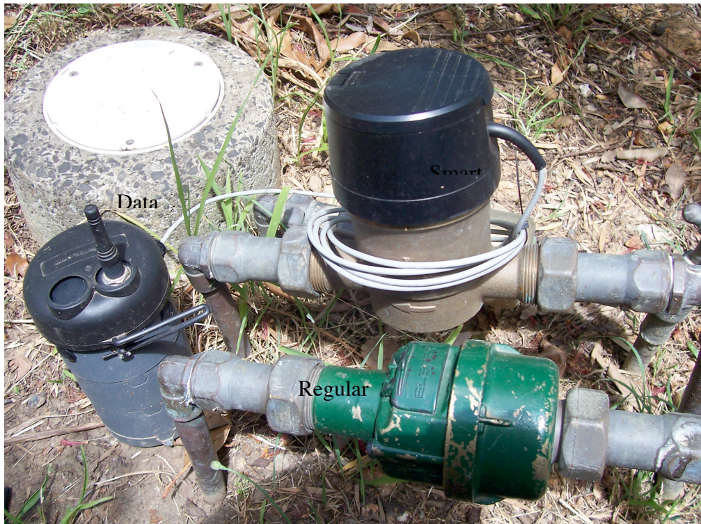
Figure 2. In-situ smart metering technology. (Source: Nicole Thornton)
