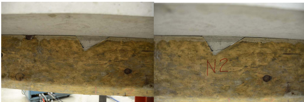
Figure 101 Connector at L/4 from the left support before (left) and after (right) failure for B-4N
