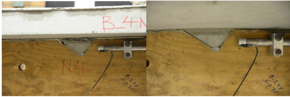
Figure 73 Connector close to the right support after the failure test (left) and before the failure test (right) for B-4N
