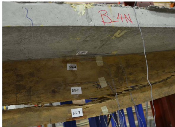
Figure 70: Tension failure of the joist B_4N
