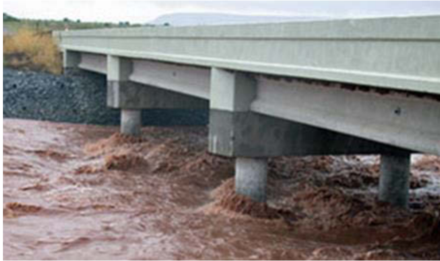
Figure 1.1 Bridge piers experiencing the flood events (USGS (2014))
