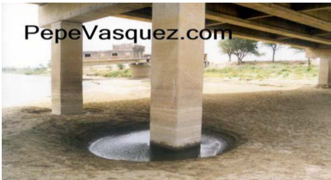
Figure 2.3 Local scour at bridge piers; (Vasquz, 2006)
