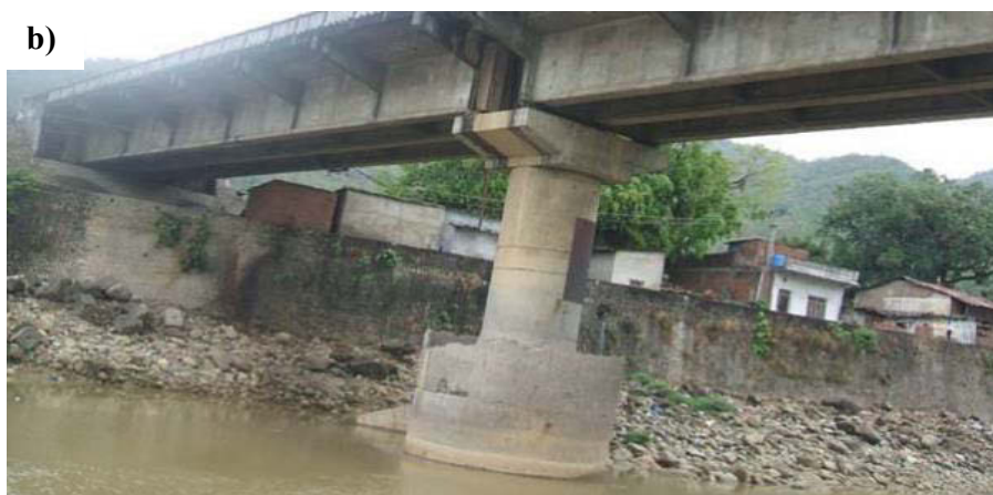
Figure 1.2 a) Scour around bridge piers on the Logan river, Australia; (Queensland Government (2013) ; and b) Scour around bridge piers on the Tinau river, Nepal, (KC (2014))
