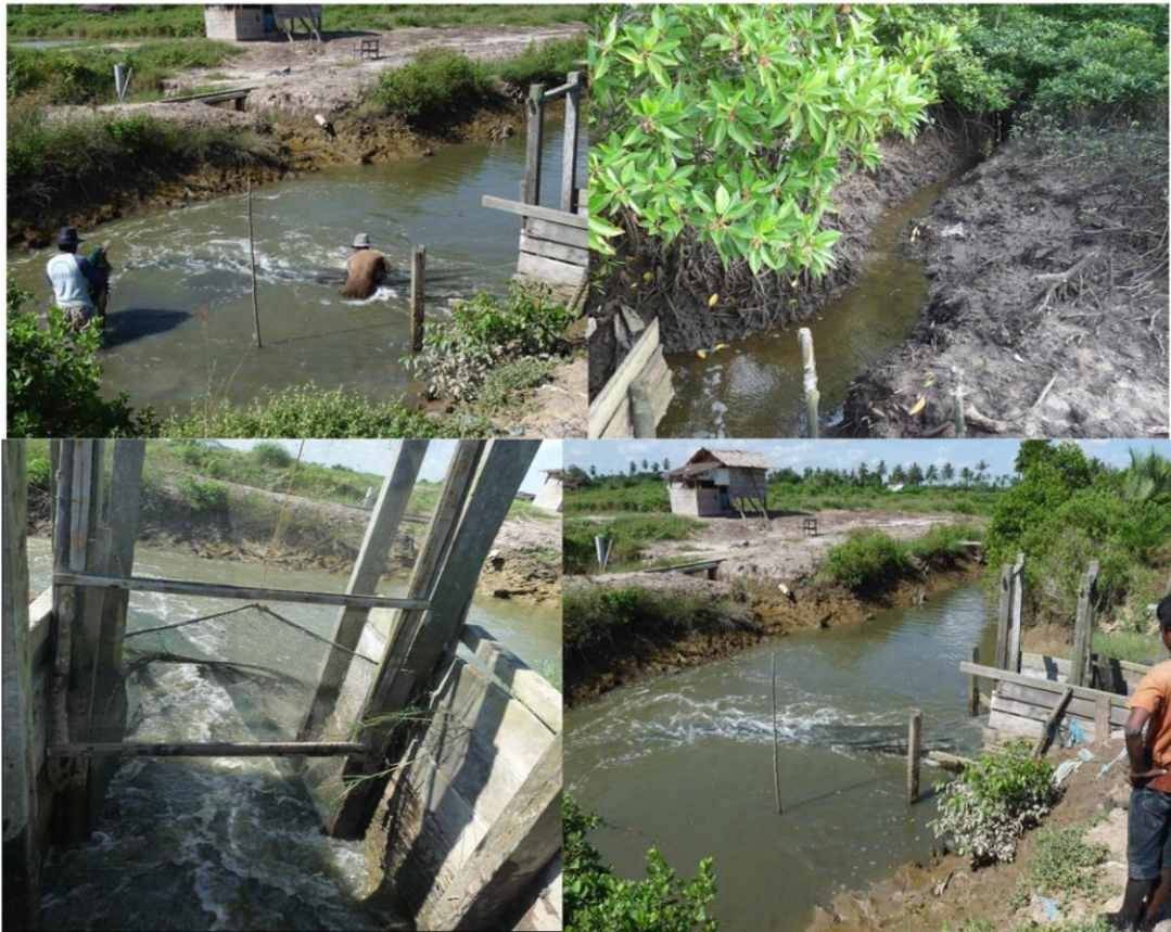
Plate 6.1 Water canal and wooden water gate for household-scale shrimp farms' water access in Aceh. The pictures show sedimentation of the water canal basin. Water access is dependent upon the tides.
