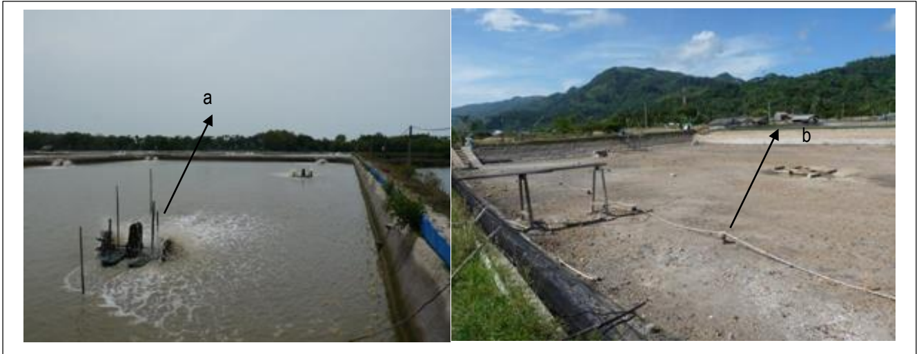
Plate 6.4 Industrial-scale shrimp ponds with concrete lining and facilitated with production facilities in Lampung; paddlewheel (a) and aerators (b).
