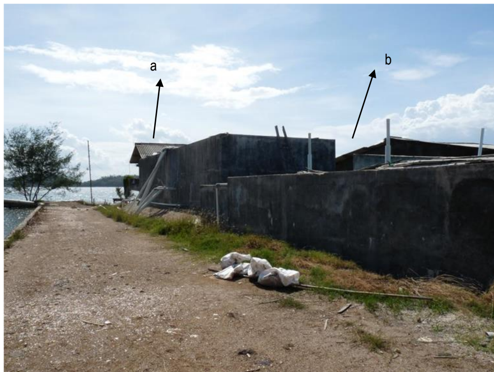
Plate 6.3 Water access facilities for industrial-scale shrimp producers in Lampung. The plate shows (a) the water pump and (b) treatment facilities. Water is sourced directly from the ocean and treated prior to distribution to ponds.
