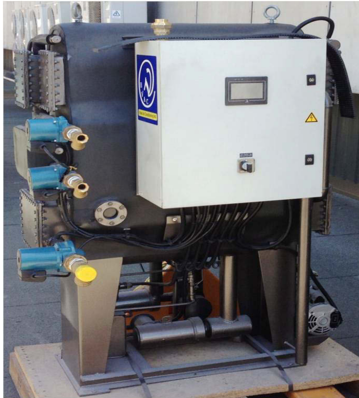
FIGURE 4.1: Viuna Absorption chiller at the top of UTS building 2
