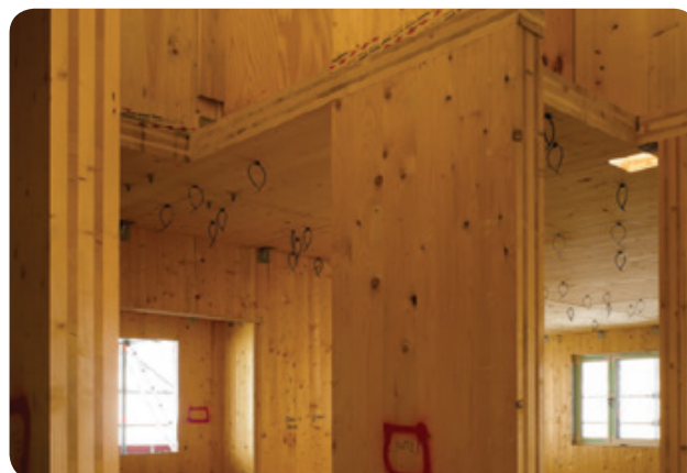
Figure 1: Cross-Laminated Timber construction
