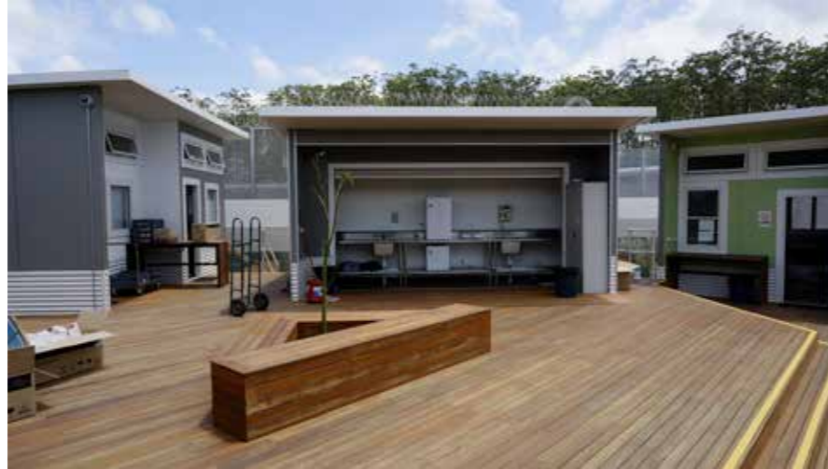
SEATING AND KITCHEN/TOILET BLOCK
