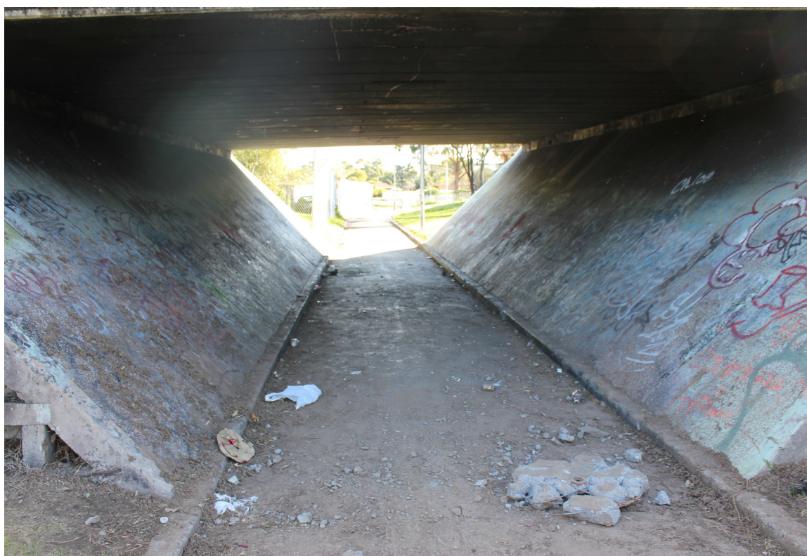
Figure 8 Existing underpass, Mt Druitt
