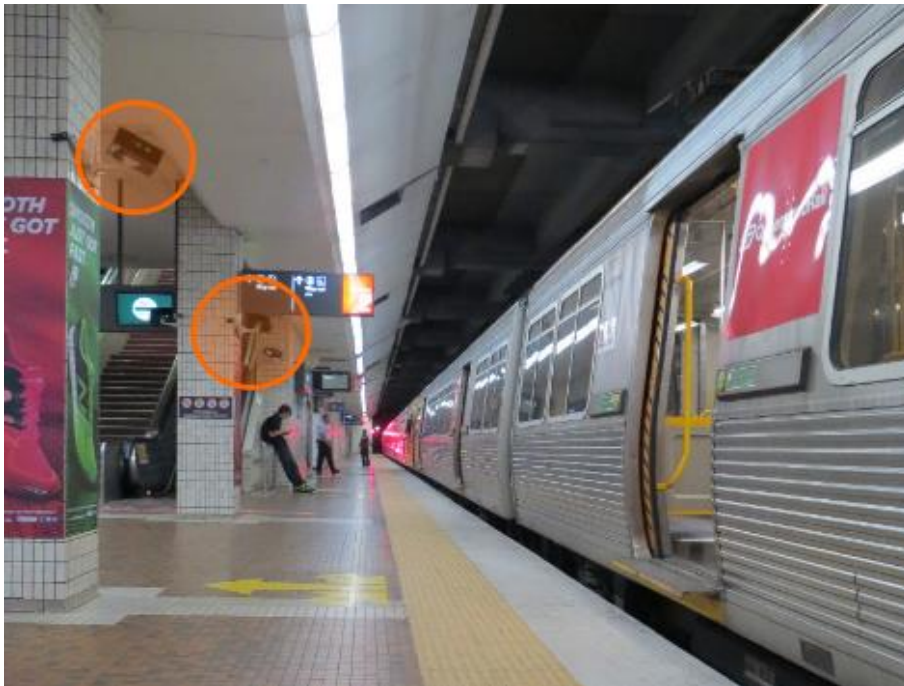
Figure 7: Picture of a 3D-RGBD sensor placed on a platform at Brisbane Central rail station.
