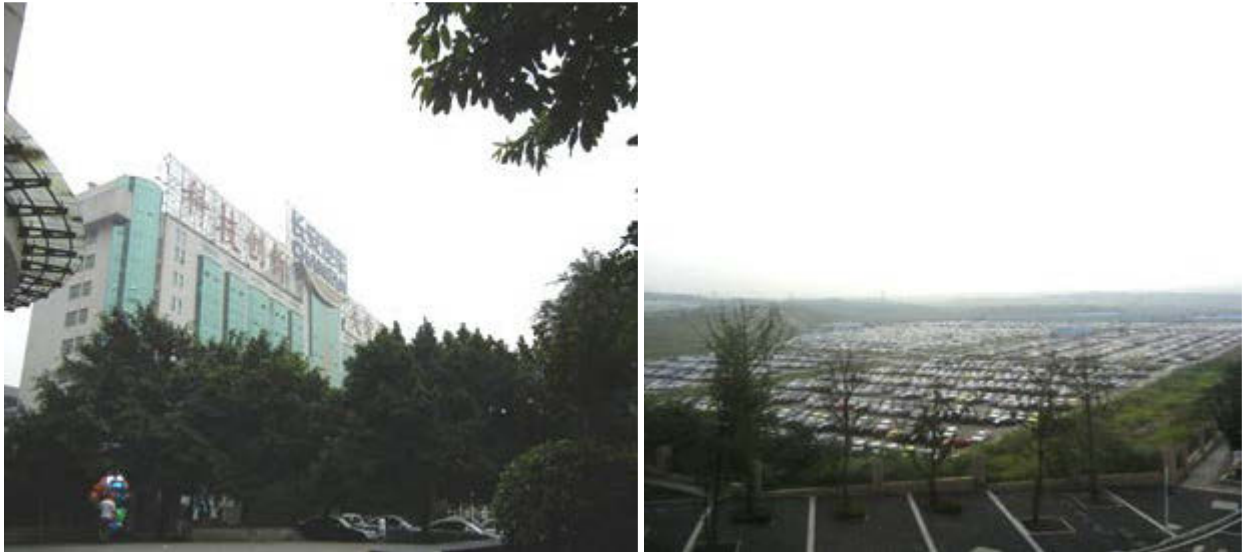
From left: Plate 6.5. The only Chang'an automobile factory in Jiangbei district. Plate 6.6. View of a parking lot full of automobiles adjacent to the Chang'an-Ford-Mazda factory in the NNZ. Photographs by the author
