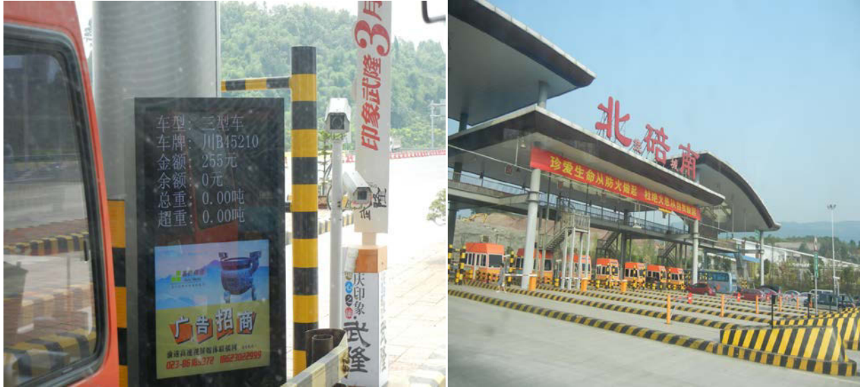
Plates 5.1 and 5.2. Toll collection points of the G75 in Beibei district.
