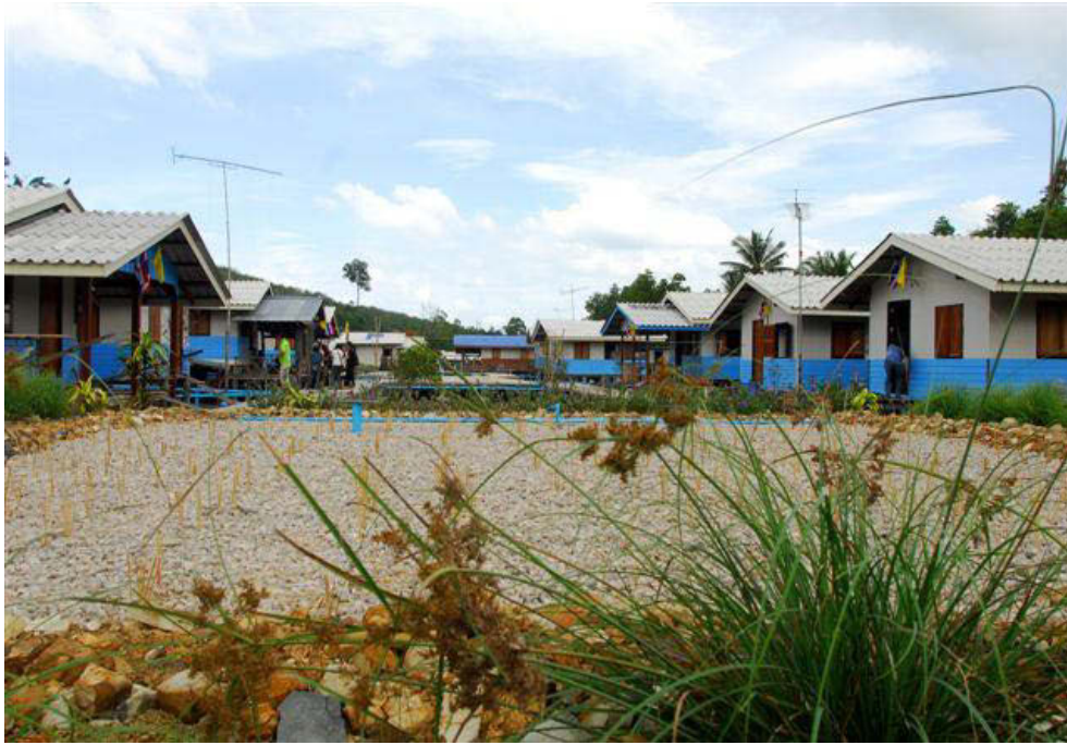
Figure 5.4: Koh Mouk Housing Project, completed in December 2007
