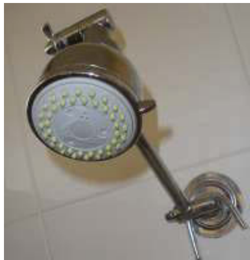
Figure 2.3 Water efficient shower heads/roses
