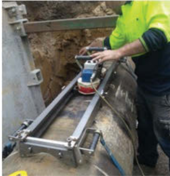
FIGURE 4.16: Industry tool on the 600mm cast iron pipe
