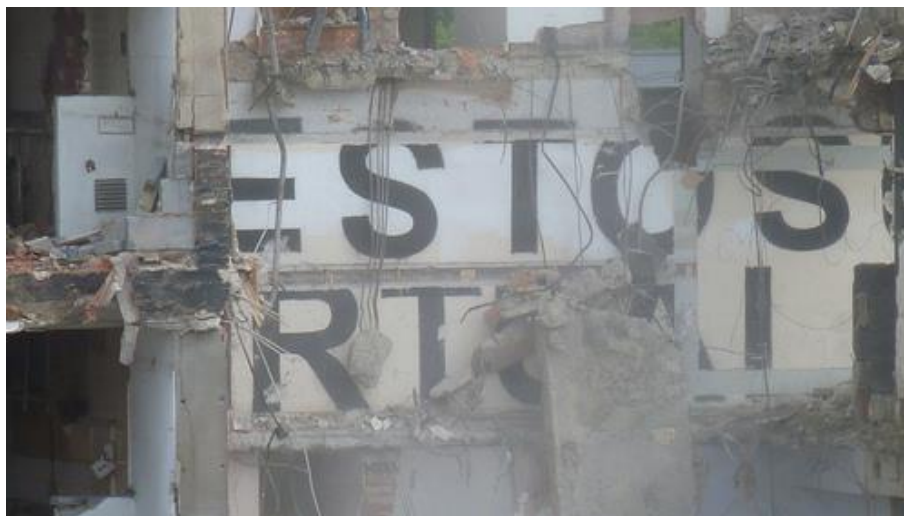
Figure 5. Detail of 'Embodied Text' during demolition
