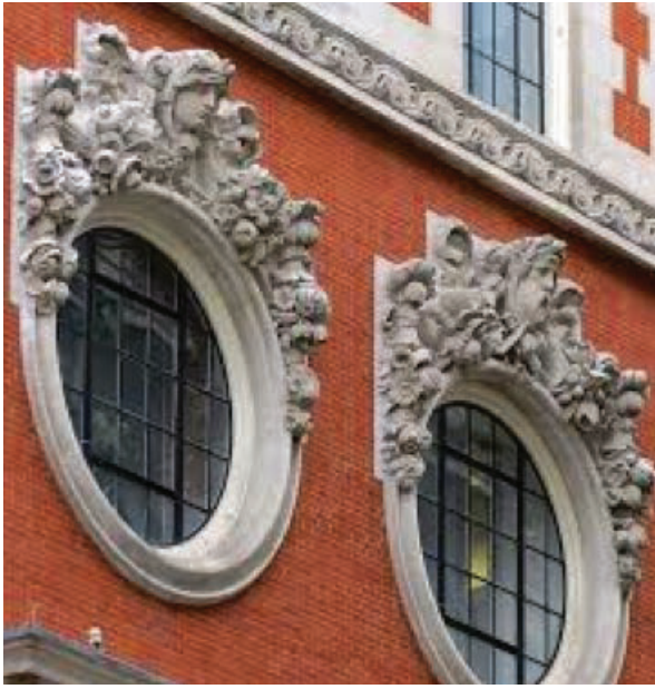
Detail of the porthole windows of the Waring and Gillows building, Oxford St, London
