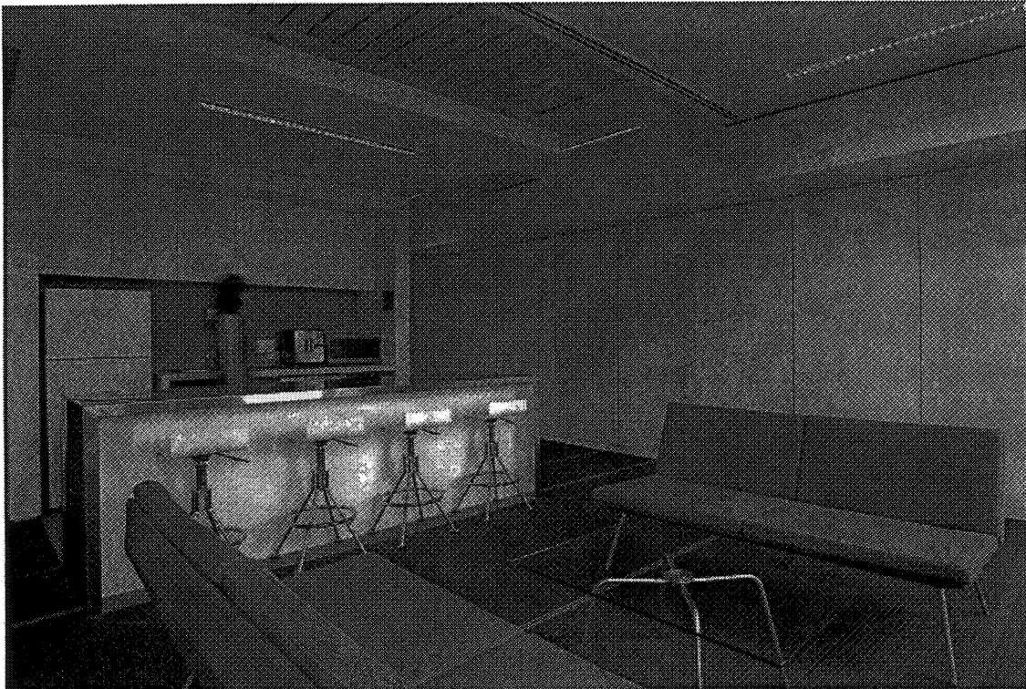
Figure 3. Staff facilities shown for Level 3 Plasterboard bulkheads band A/C ducts and structure together, exposing the thermal mass of the slab above.
