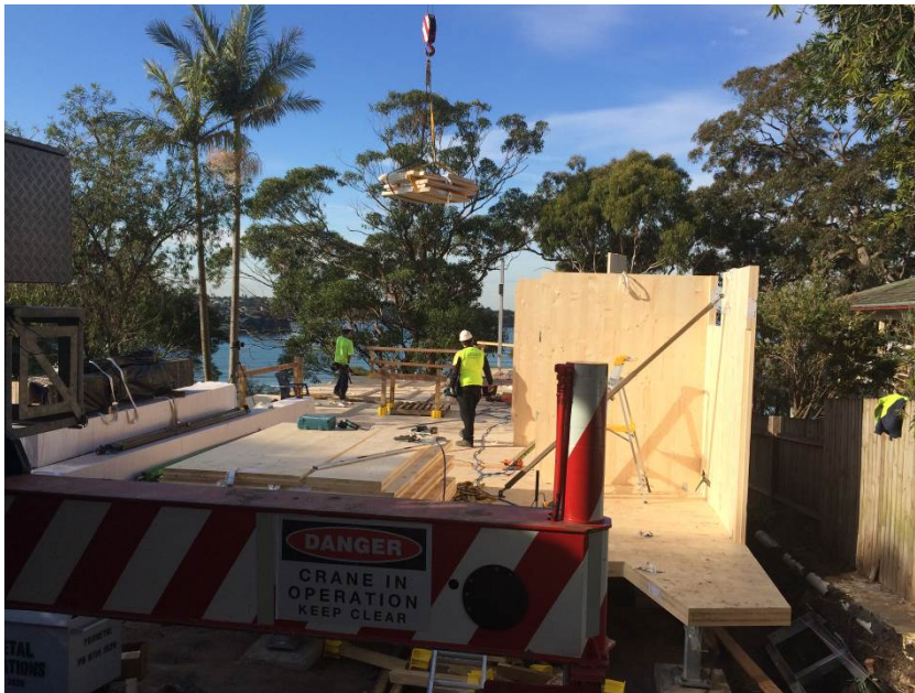
Figure 3: Panels being manoeuvred into position.
