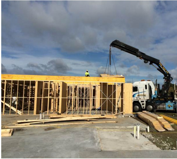
Figure 4: Floor cassettes during installation.
