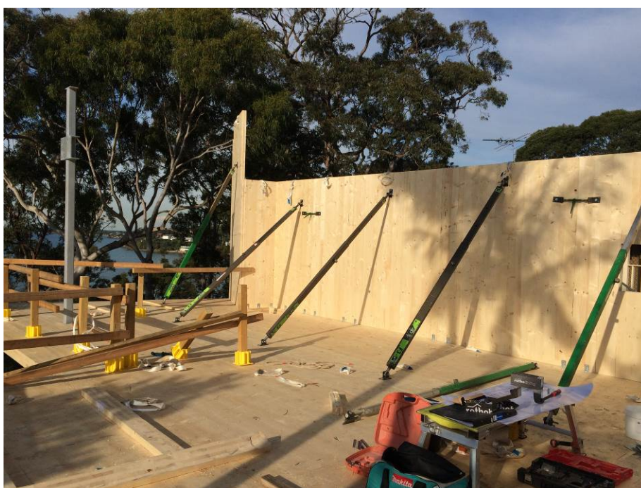
Figure 2: Cross Laminated Timber wall temporarily panels braced during construction.
