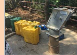
Privately operated metered handpumps, Uganda
