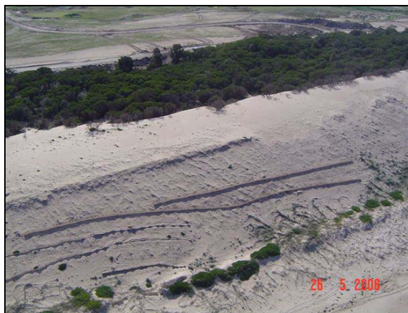
Figure 6. Placement of jute fencing.
