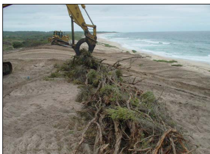
Figure 7. Coastal tea-tree being placed on the reconstructed dune crest.
