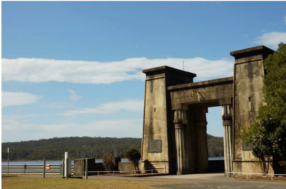
Figure 9: Location Photograph - Cataract Dam
