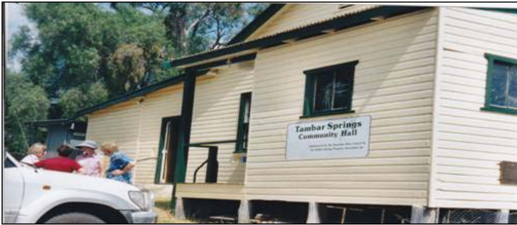
The Tambar Springs Community Hall (Source: Foster, J, April 1, 2003)
