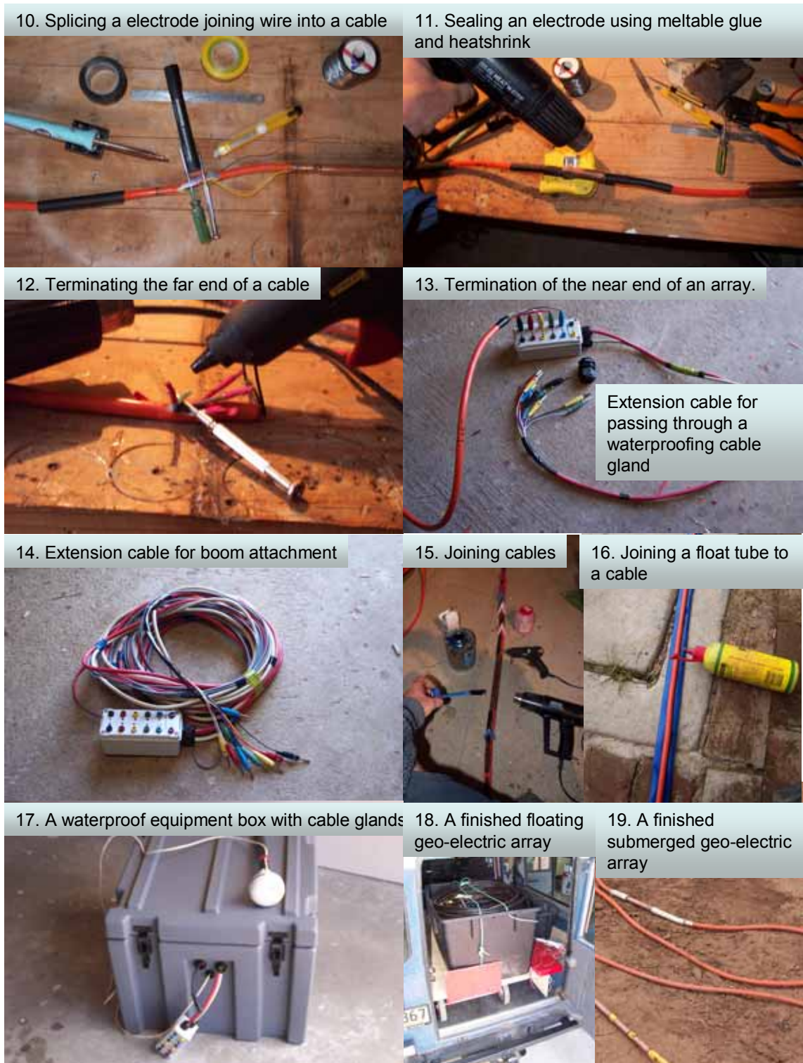
Figure A1-2 Towed geo-electric array construction, part 2.
