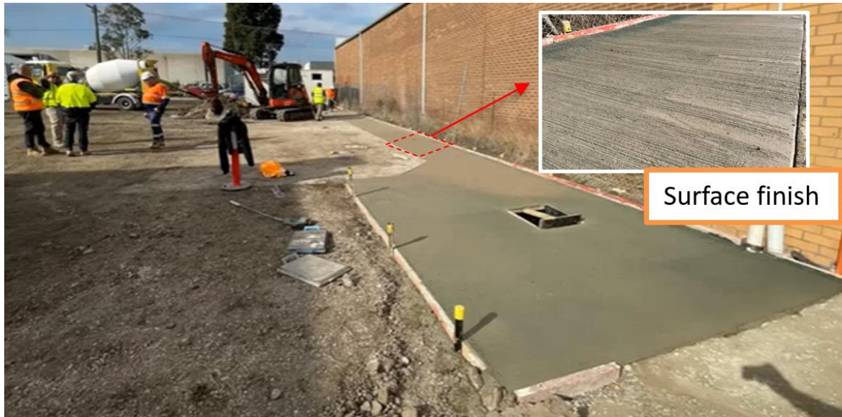
Figure 4 GPC footpath placement and finished surface texture
