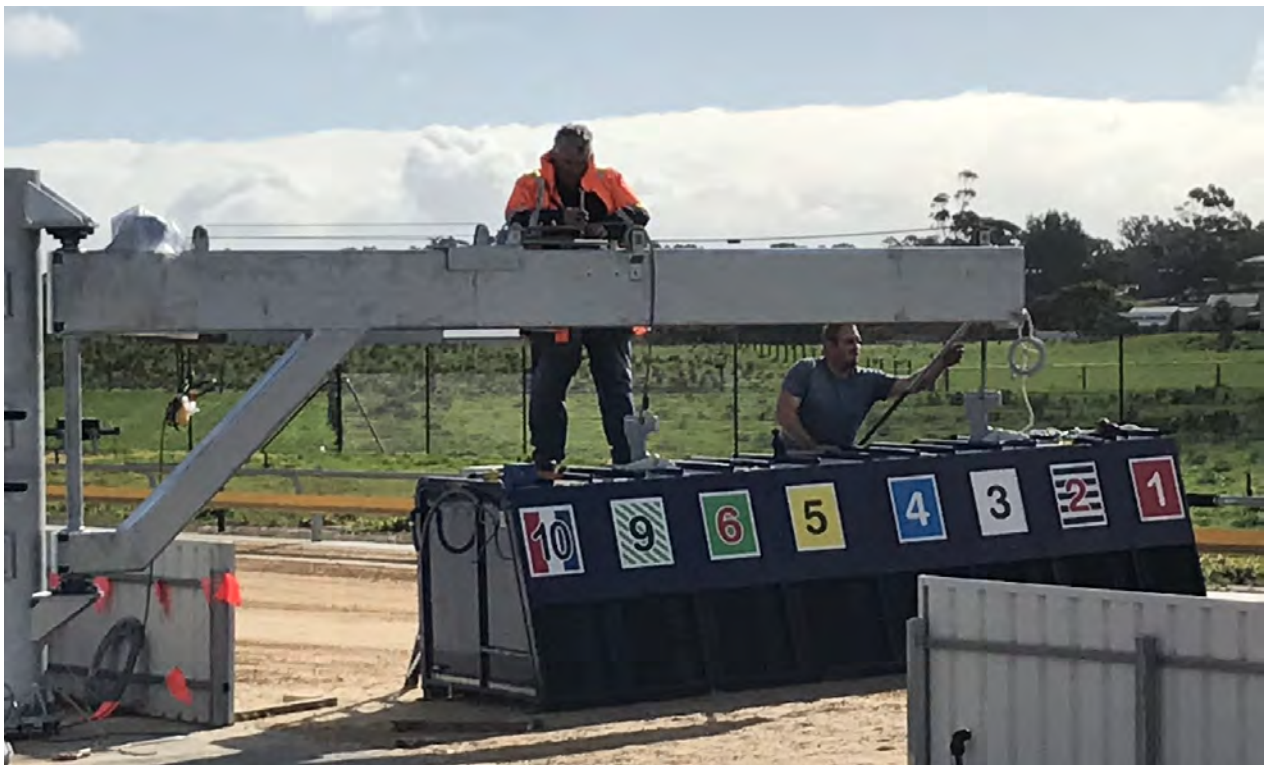
Figure 14: Murray Bridge drop-on boxes being installed (11 July 2019.)
